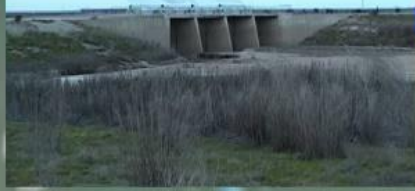
Chowchilla Bypass Structure
