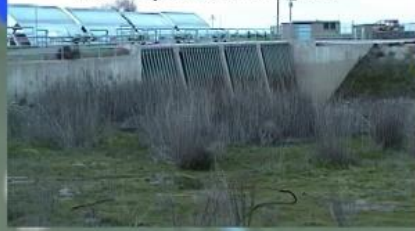
San Joaquin River Structure
