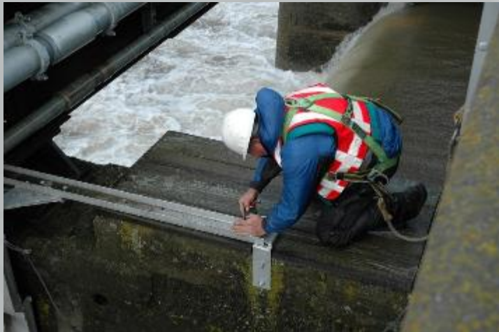
Photo: DWR Flood Maintenance Office Employee Opening One Bay of the 100-year old Sacramento Weir during the winter 2017 high water event. The weir protects the cities of Sacramento, West Sacramento and Elk Grove by removing flood flows from capacity limited Sacramento River.
