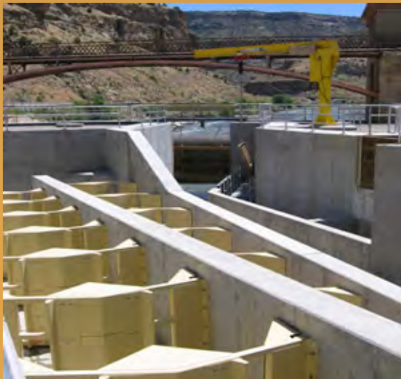
A fish passage at the Grand Valley Project Diversion Dam on the Colorado River provides endangered fish with access to critical habitat in western Colorado. Source: Bureau of Reclamation
