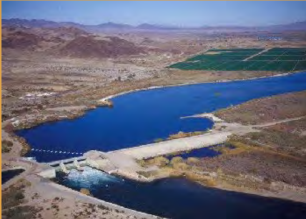
Palo Verde Diversion Dam Source: Bureau of Reclamation
