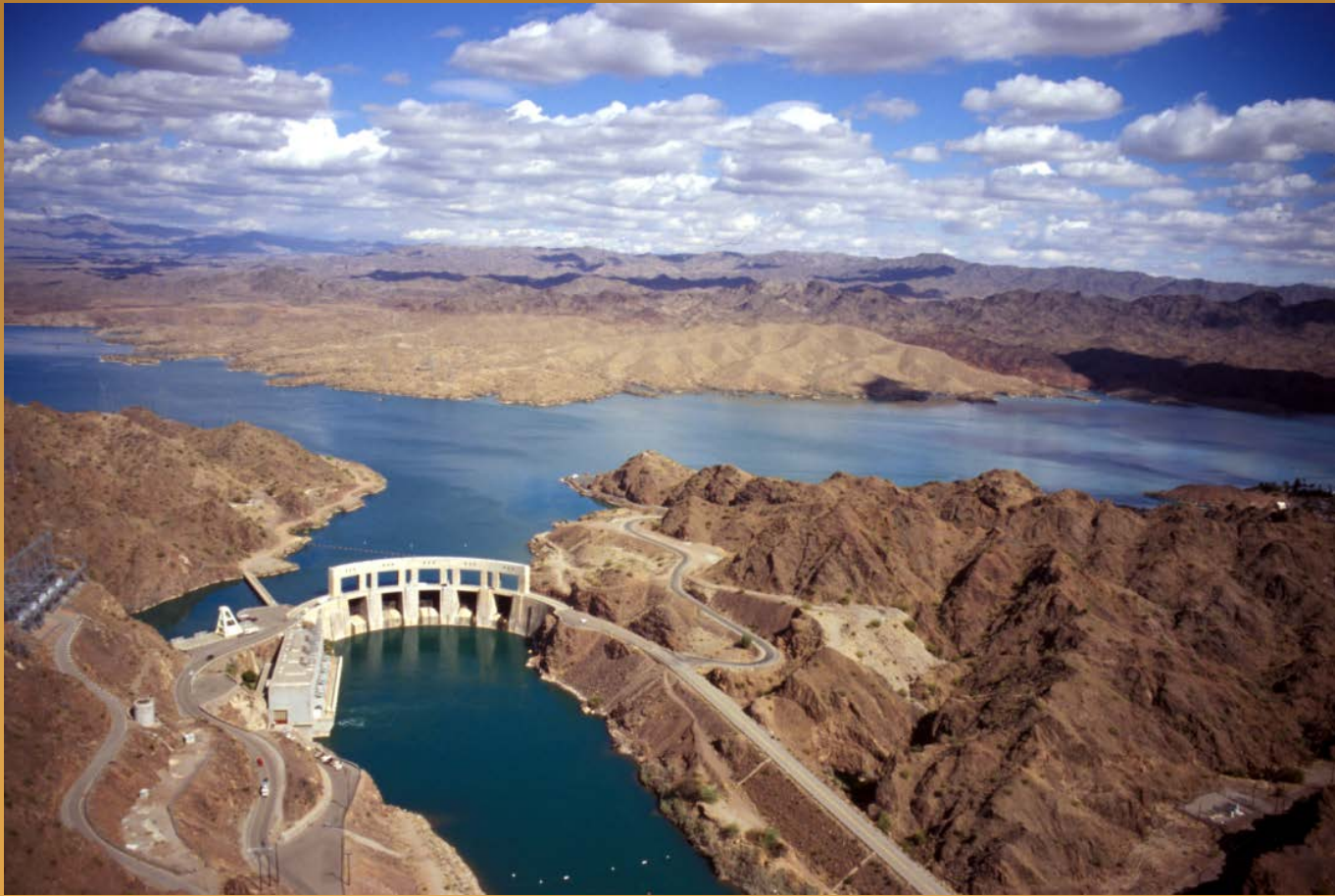
Parker Dam where water is initially drawn into Colorado Aqueduct
