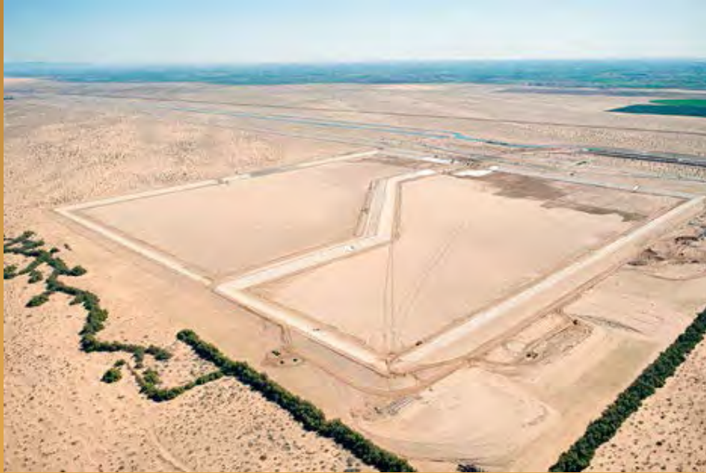
Brock Reservoir construction Source: Bureau of Reclamation
