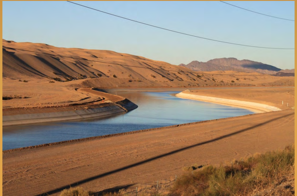
The All-American Canal – built between 1934 and 1940 – stretches 80 miles through the Colorado Desert to Southern California and is part of the federal irrigation system from the Hoover Dam.
