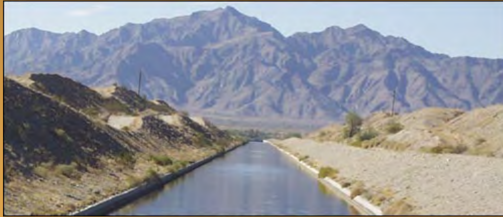
Wellton-Mohawk Main Canal Source: Wellton-Mohawk Irrigation and Drainage District
