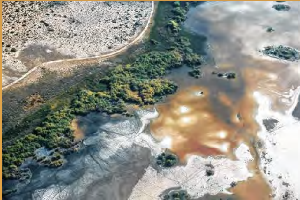
The Gila River flooded and damaged the desalting plant in 2003.
