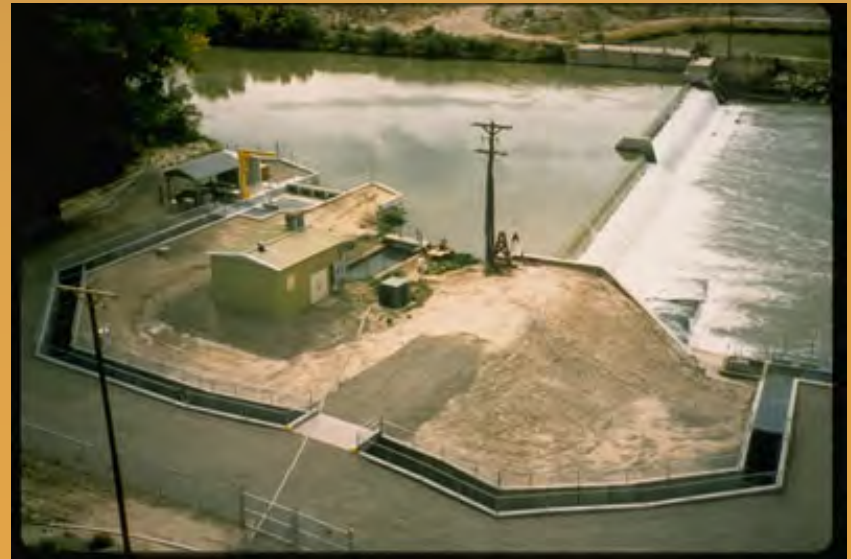
The fish ladder installed in 1996 at the Redlands Diversion Dam near the mouth of the Gunnison River allows upstream passage of native fishes and aids in recovery of endangered Colorado pikeminnow and razorback sucker populations. Source: Bureau of Reclamation
