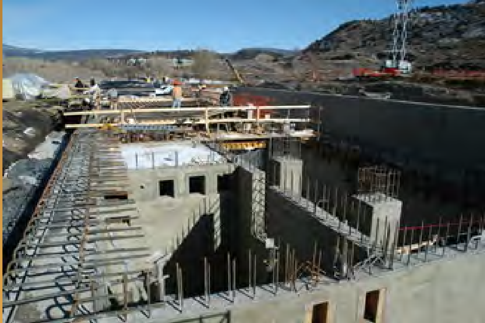
Animas-La Plata construction. Source: Bureau of Reclamation
