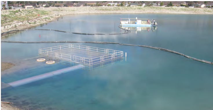
FIGURE 8: OCWD GROUNDWATER RECHARGE SITE (SOURCE: OCWD)
