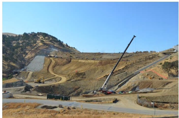
FIGURE 5: LOS VAQUEROS DAM DURING CONSTRUCTION - SUMMER 2011
