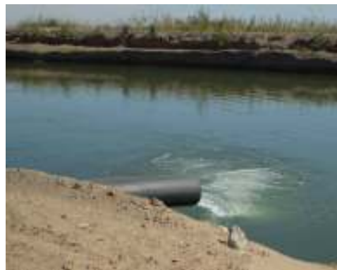
Seepage water pumped from the EHL 14 Drain flows into the East Highline Canal
