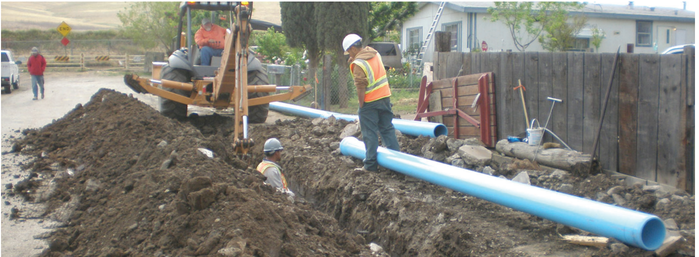
Photo caption. Grant funding is used to improve water system connectivity.
