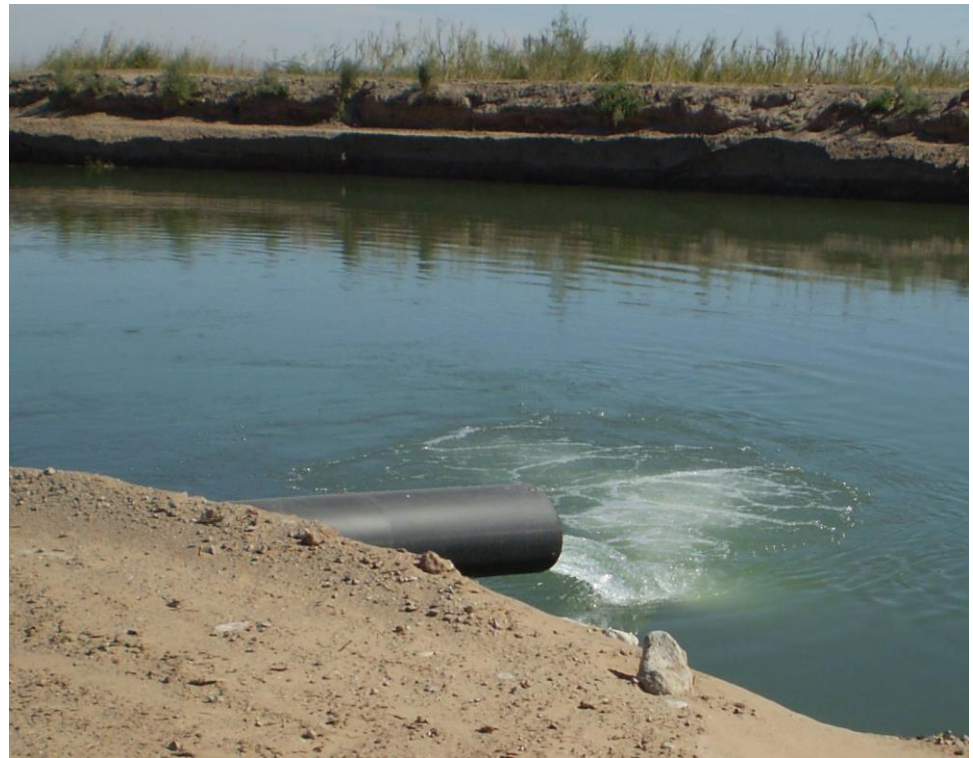
Seepage water pumped from the EHL 14 Drain flows into the East Highline Canal
