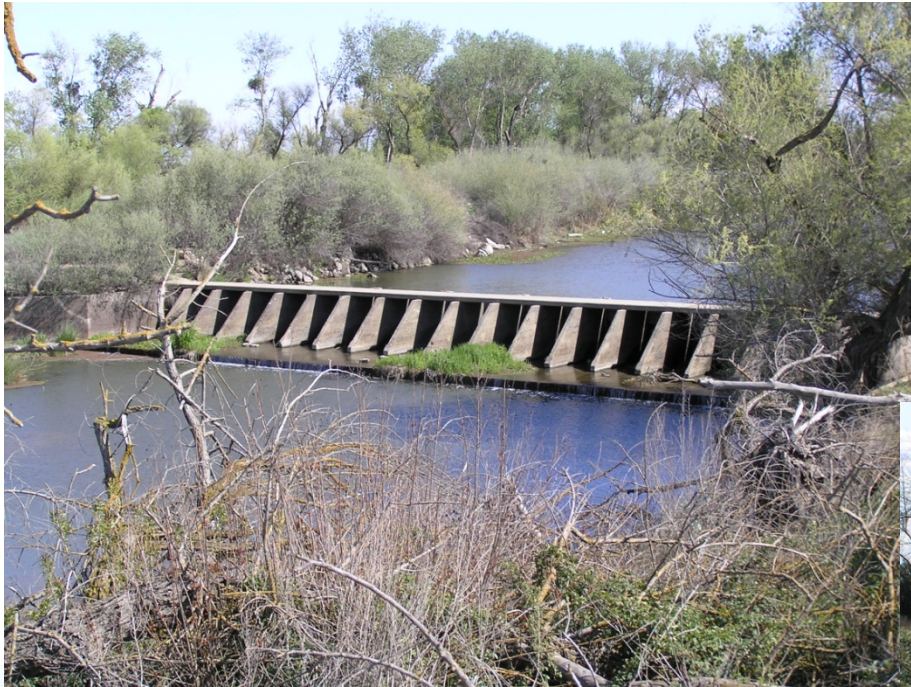
Sack Dam – Modify for fish passage
